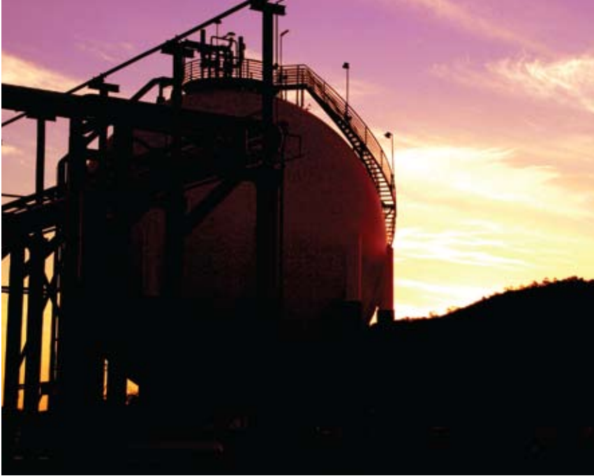
◀ Sphere for Liquefied Petrol Gas (LGB) storage.
