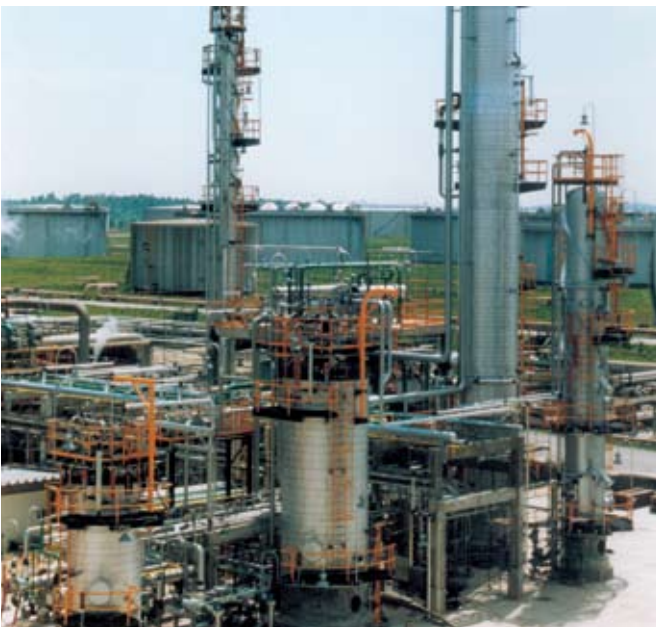
▼ MTBE system – capacity 79,000 ton/yr.
